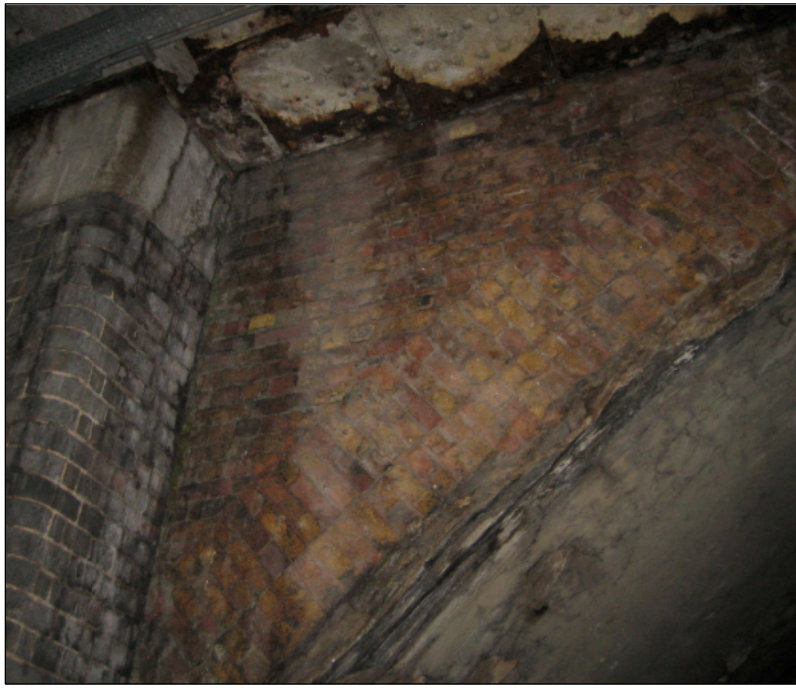
EXAMPLES OF DEGRADATION OF JACK ARCH BEAMS DUE TO WATER INGRESS FROM PARK LEVEL ABOVE - Please see Structural engineers report for description of required remedial works.
